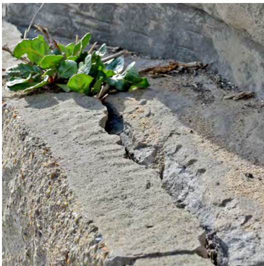
5.25: OPEN JOINT TO BLOCK PLINTH (A08)
