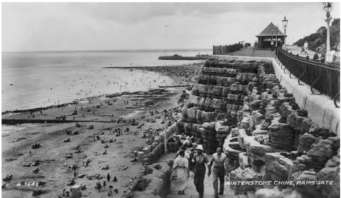
4.08: EAST CLIFF CHINE SOON AFTER OPENING (NOTE LACK OF PLANTING)
