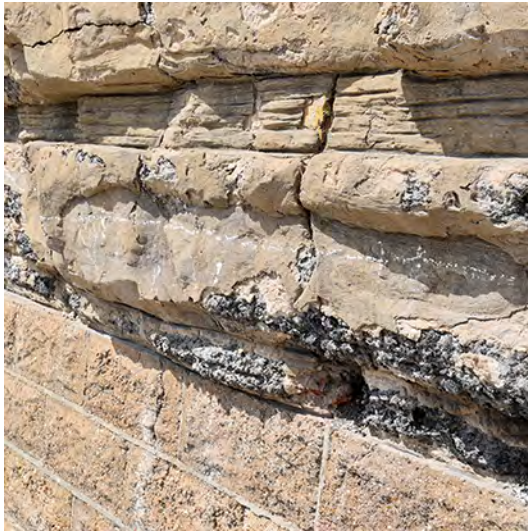
2.23: CONCRETE BLOCK BACKING
