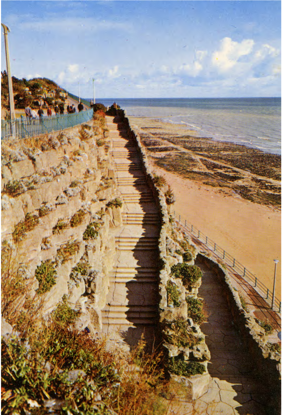
4.09: LOOKING DOWN ONTO TOP FLIGHT OF THE CHINE SHOWING ROWS OF PLANTERS (ASSUMED — ON BASIS OF CONCRETE LAMP POST — 1950s or 1960s)
