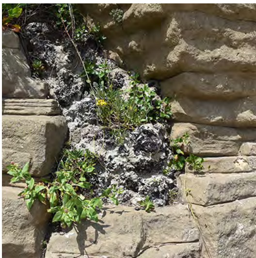
2.25: BURRS PACKED INTO FISSUE
