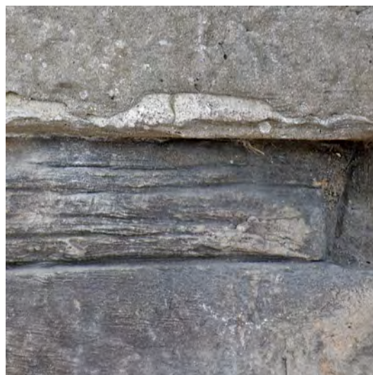
5.02: MINIMAL RAIN WASHING PERMITS BUILD-UP OF AIRBORNE DIRT (A10)
