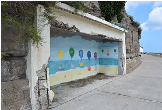
2.13: REINFORCED CONCRETE SHELTER
