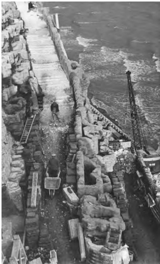
4.01: UNDER CONSTRUCTION 1936 (NOTE CHUTE NEAR CENTRE RIGHT)
