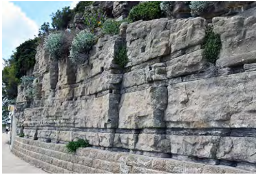
2.11: GENERAL VIEW OF LOWER FACE
