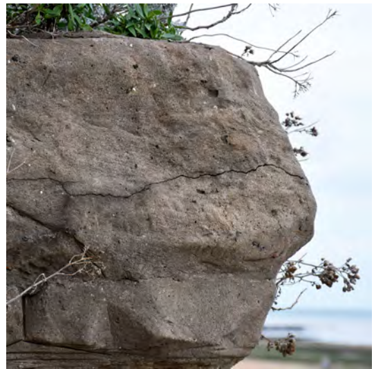
5.14: HAIRLINE FRACTURE (A11A)
