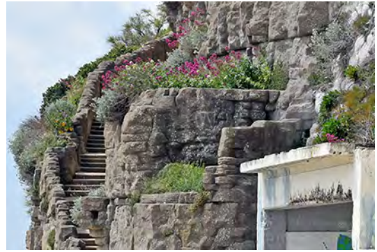
2.12: ROCKWORK AT NORTHERN END
