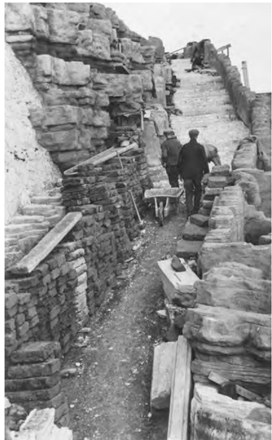
4.02: UNDER CONSTRUCTION 1936 (NOTE CONCRETE BLOCK BACKING)
