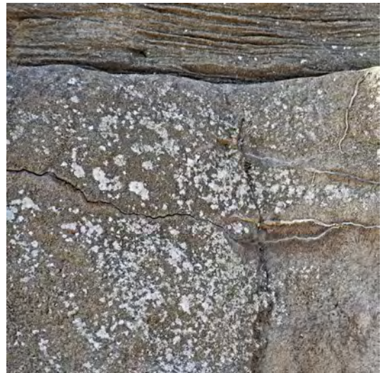
5.18: CRYSTALLINE VEINS + CRACK (A05)
