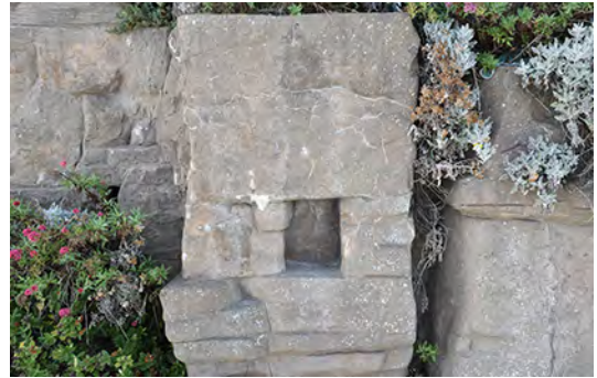
4.04: ASSUMED EXIT OF CHUTE FOR DELIVERY OF CONCRETE
