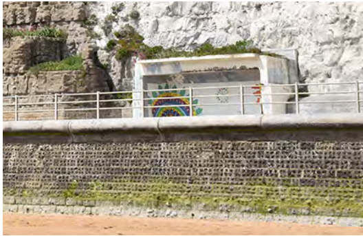
4.03: FLINT-FACED SEA WALL & CONCRETE SHELTER
