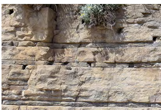
2.09: CLOSE-UP SHOWING PUTLOGS
