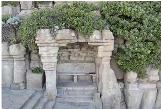
2.19: SHELTER NEAR END OF MIDDLE FACE
