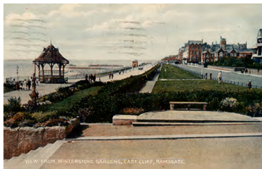
4.06: LOOKING SOUTHWEST ALONG EAST CLIFF BEFORE 1935 (COMPARE 4.08)
