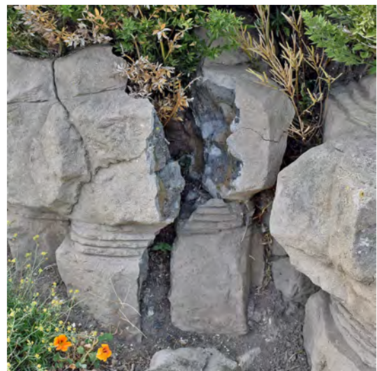
5.20: FRACTURE & DISPLACEMENT (A10)
