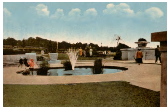
4.07: POOL, FOUNTAIN & SEAT BEFORE 1931 (NO HOUSES ON WINTERSTOKE CRESCENT)
