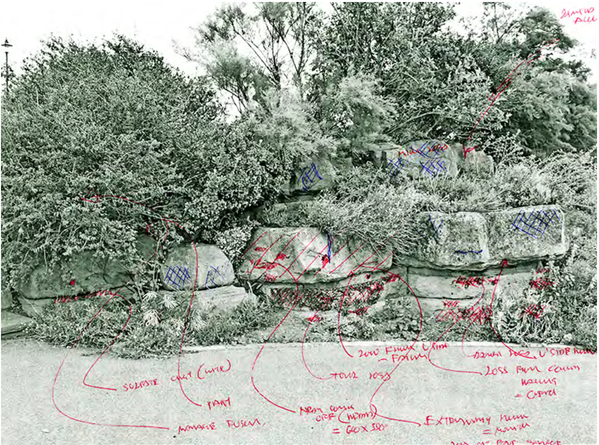
BASE SURVEY PHOTO (TOP) & MARKED-UP COPY (BOTTOM)
