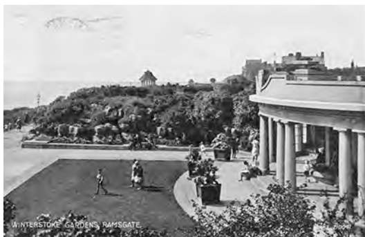
4.03: LOOKING SOUTHWEST ACROSS SUN SHELTER (BEFORE 1935; PC DATED 1948)
