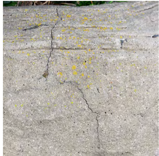
5.18: HAIRLINE FRACTURE (A14A)
