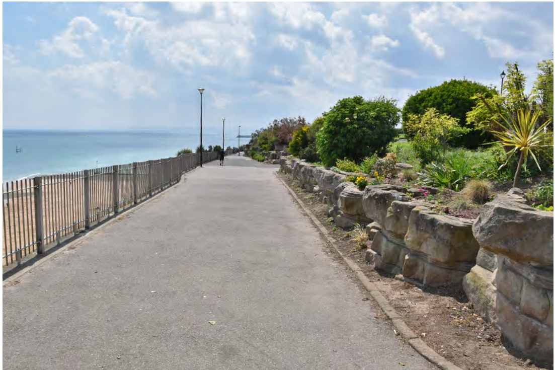
2.06: THE ROCKWORK OF WINTERSTOKE GARDENS (RIGHT) STRETCHING ALONG THE CLIFFTOP PROMENADE
