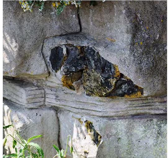
2.16: BRICKS AT BASE OF PLANT POCKET
