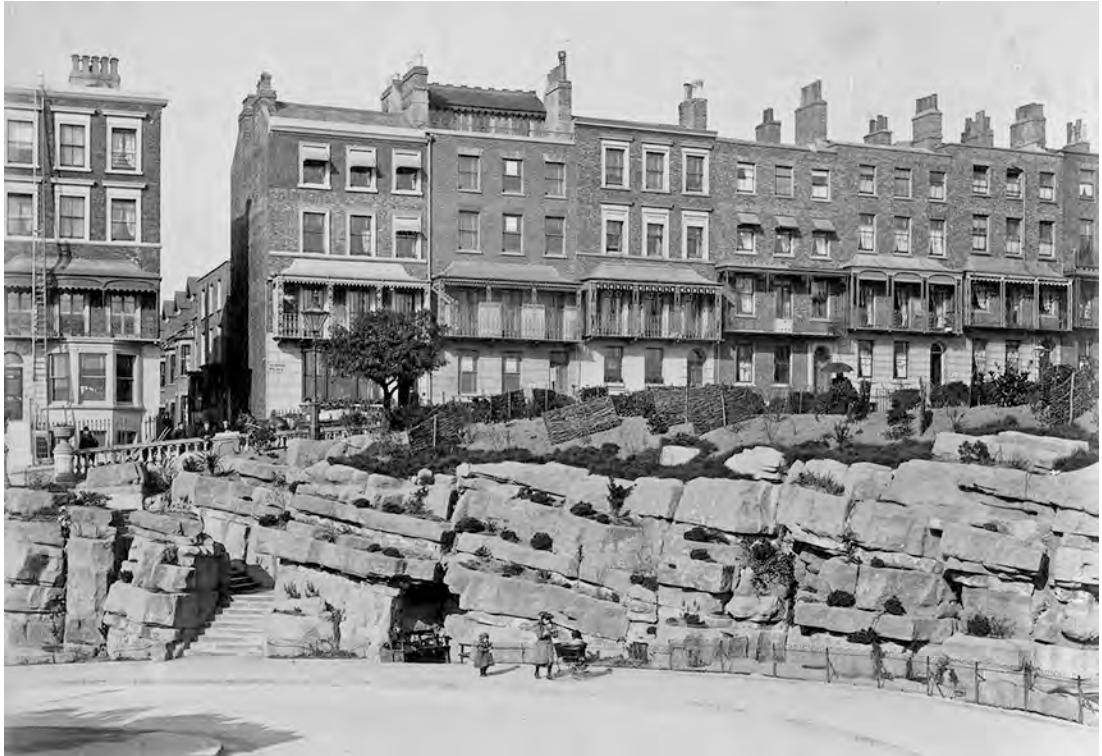
4.05: NORTH SIDE OF MADEIRA WALK SOON AFTER COMPLETION IN 1894 — NOTE RECENT PLANTING & TEMPORARY HURDLES
