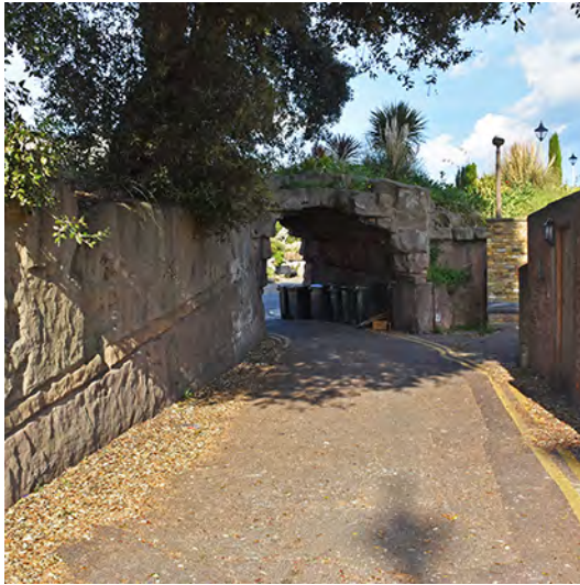
2.29: ROADWAY &amp; REAR OF ‘TUNNEL’
