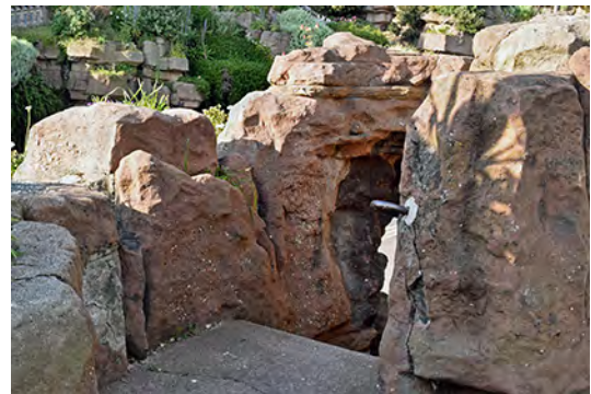
2.26: CRUDE ROCK ARCH OVER STAIRWAY
