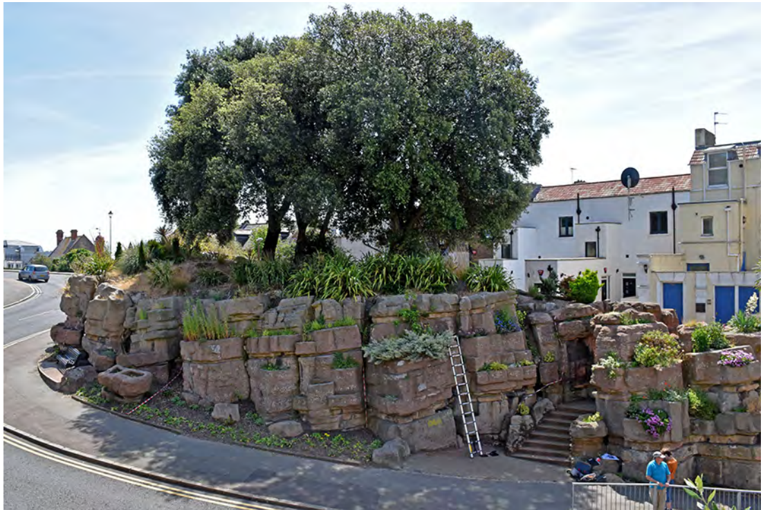
2.24: SECOND (CENTRAL) SECTION OF SOUTH SIDE OF MADEIRA WALK
