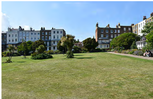
2.02: ALBION PLACE GARDENS WITH REGENCY TERRACES OF ALBION PLACE
