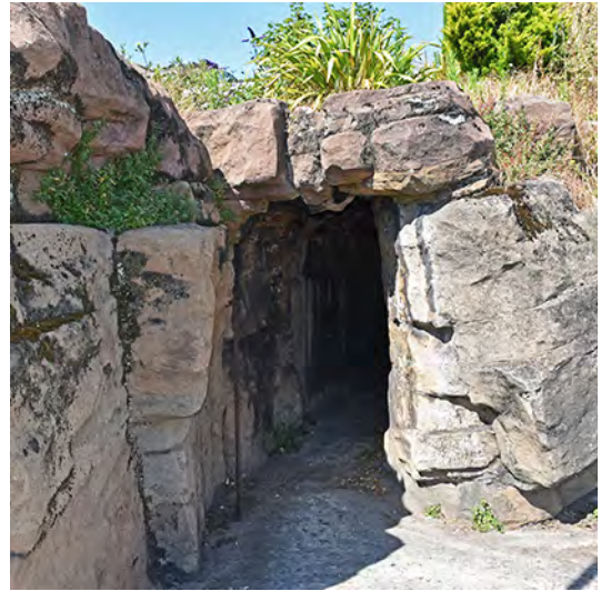
2.30: PASSAGEWAY TO REAR OF OAK HOTEL
