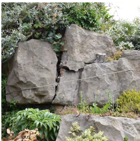
5.21: FRACTURE &amp; COLLAPSE (N29)
