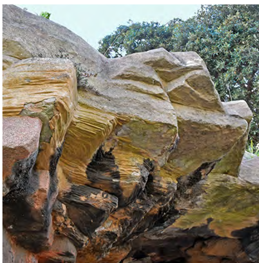
2.35: CANTILEVERED STONE SLABS CORBEL TO FORM ROOF OF TUNNEL
