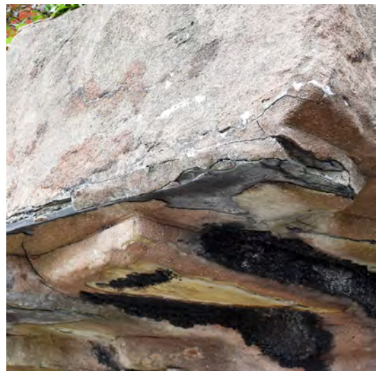
5.10: UNDERSIDE LOSS (N16)
