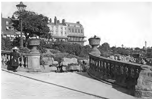
4.06: VIEW FROM ALBION HILL (BALUSTRADE INTACT) BEFORE 1901 (HEA ref. OP00657)
