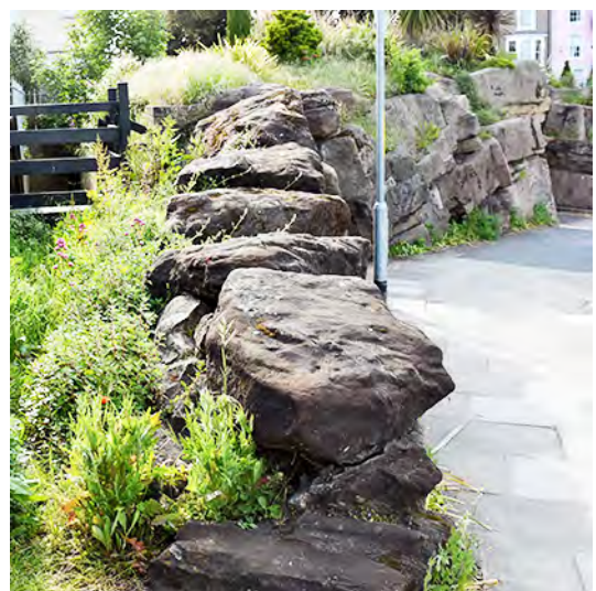
2.36: SANDSTONE BOULDER COPING TO PAR ON SOUTH SIDE OF MADEIRA WALK
