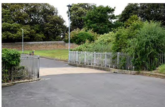
2.02: BRIDGE CARRYING END OF WEST CLIFF PROMENADE OVER THE CHINE
