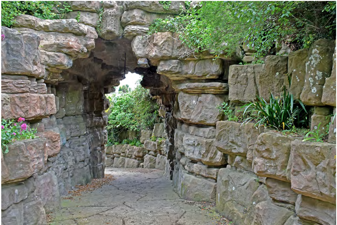
2.06: PAR 'TUNNEL' (ARCH) PASSING UNDER THE CLIFF PROMENADE (SEE FIG. 2.02)
