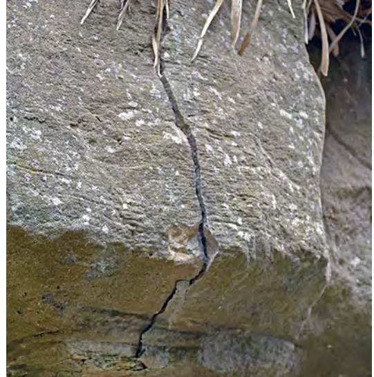
5.12: FULL-HEIGHT FRACTURE OF PLANT POCKET & OVERHANG
