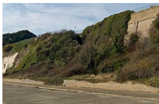
2.03: WESTERN UNDERCLIFF WITH CHINE (ABOVE) & CONCRETE RETAINING WALL
