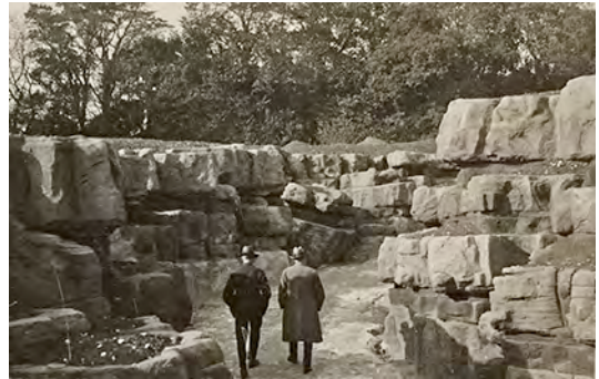
4.05: INSPECTION OF THE CHINE ON 23RD OCTOBER 1928 (KA ref. FO/S1/98/1)
