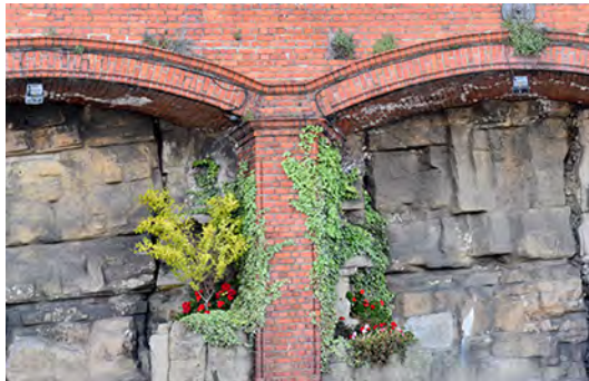
2.09: CONTINUOUS STRATA (BAYS 04 & 05)
