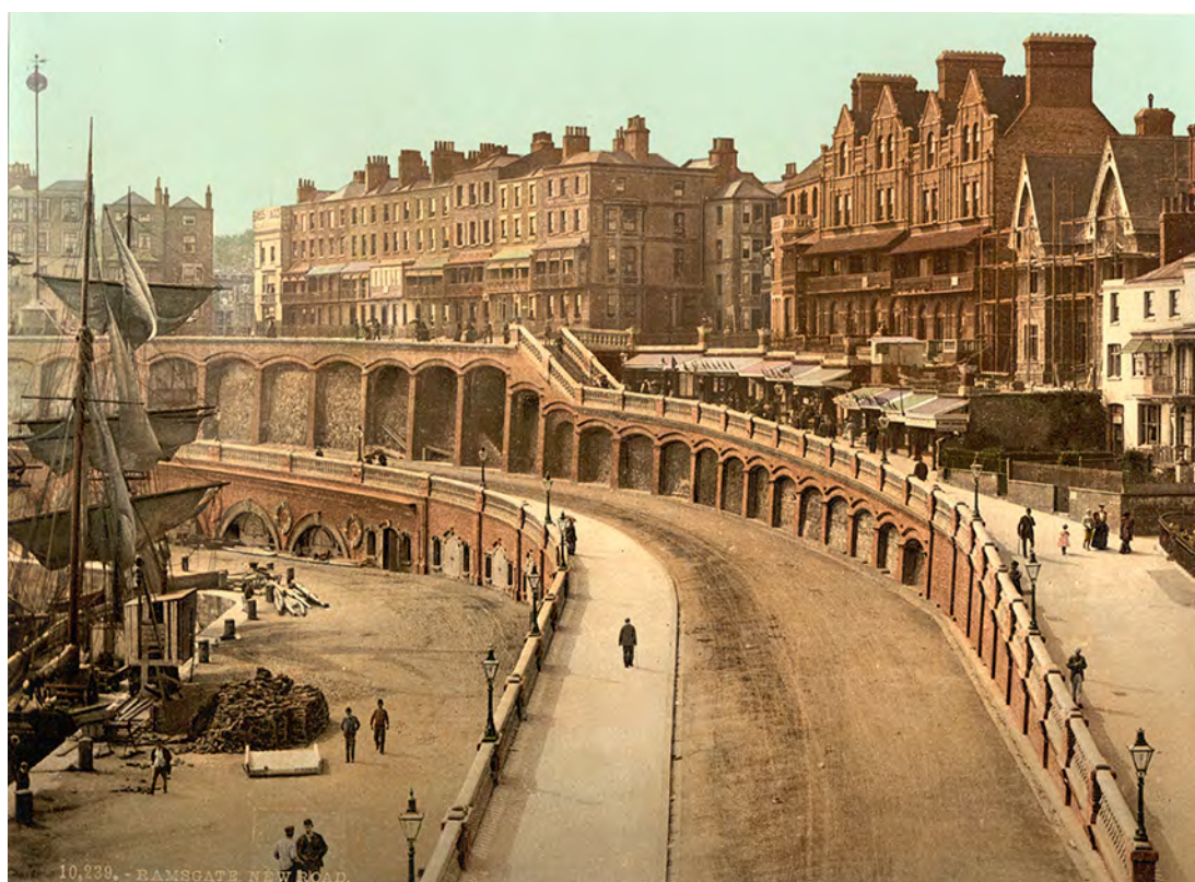
4.02: ROYAL PARADE AFTER COMPLETION IN 1894 BUT BEFORE FILLING OF ARCHES WITH PAR IN 1895 (LOC ref. LOT 13415, no. 825)
