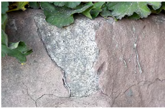
2.15: GRANITE USED IN BACKING (BAY 17)
