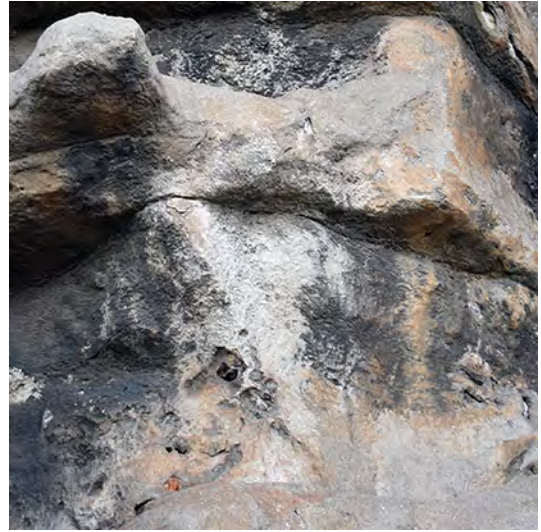
5.02: SURFACE EFFLORESCENCE
