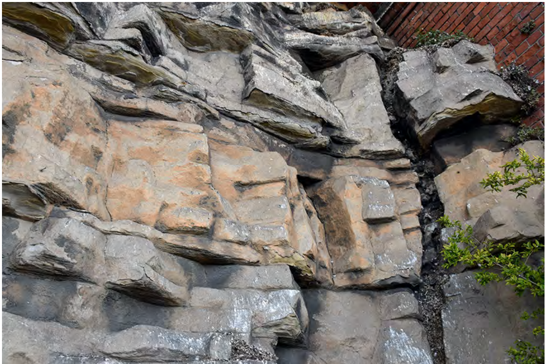
2.17: TYPICAL 'DEEP BAY' ROCKWORK (BAY 15)
