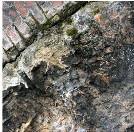
5.06: INTERACTION BETWEEN AIRBORNE DIRT & SULFATE CRUSTS
