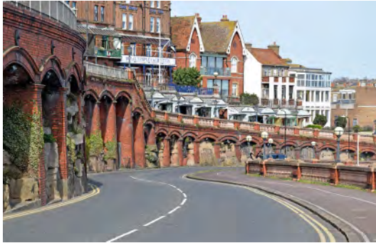
2.02: LOOKING EAST DOWN ROYAL PARADE (WEST CLIFF ARCADE ABOVE)
